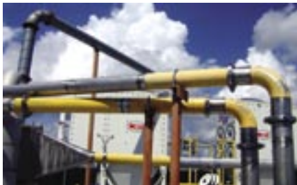
Solvay paints Conforma Clad® components yellow to distinguish them from unprotected piping.
